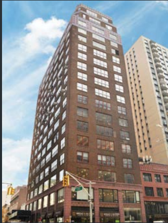
419 Park Avenue South
